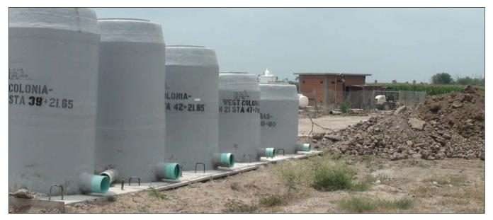
Sanitary sewer manholes to be installed with new lift station in the background, in La Feria TX
