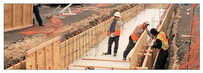
Construction of a bioretention basin at Ramsey Park, parking lot to collect and treat stormwater runoff
